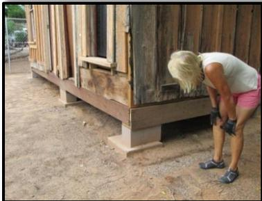
*Upper left:* The historic landmark is now level and on a firm footing. Later, a new façade will replace the peaked roof overhang and a porch will be added.
