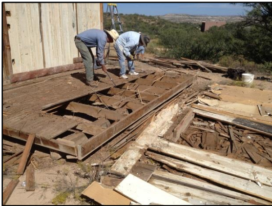
Top: Tearing up flooring & removing a room; sorting, piling, pulling nails and preserving reusable materials. Left: Disturbing roof mouse habitat. Right: Mixing cement & pouring footers .
